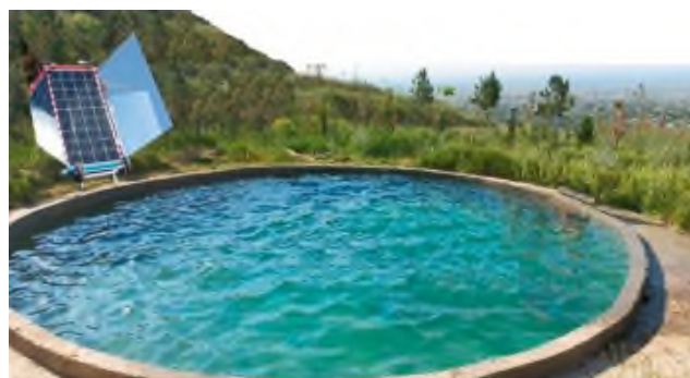
Fig. 3. A pool with a volume of 80 m 3 and a photovoltaic system for drip irrigation.
